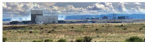
Columbia Generating Station
